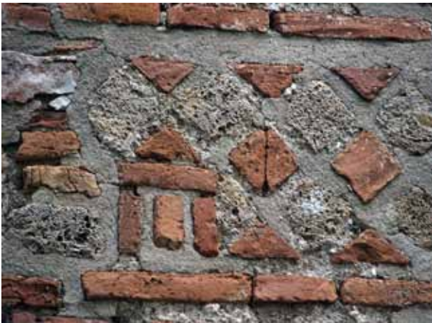
Fig. 6. Brick arrangement at southern facade, Zaum church, photo: Jasmina S. Ćirić
